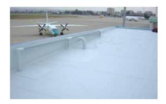
It is the soft PVC water membrane attached with hot air welding, resistant to atmospheric conditions and solar rays, polyester reinforced. The Multiplan FG serial PVC Multiplan's Water Insulation Membranes, are developed especially for all the roofs that are exposed to severe weather conditions and solar rays.
