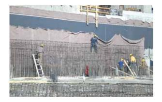
Multiplan BA is a soft PVC water insulation membranes that are with UV non-resistance, non-reinforced, welded with hot air, may be used at the foundation bundling and in the covered water insulation details.
