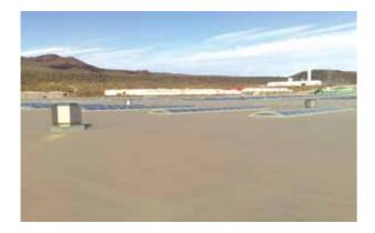
Soft PVC water membranes that are geo textile felt laminated, welded with hot air are resistant to atmospheric conditions and solar rays, polyester reinforced.
